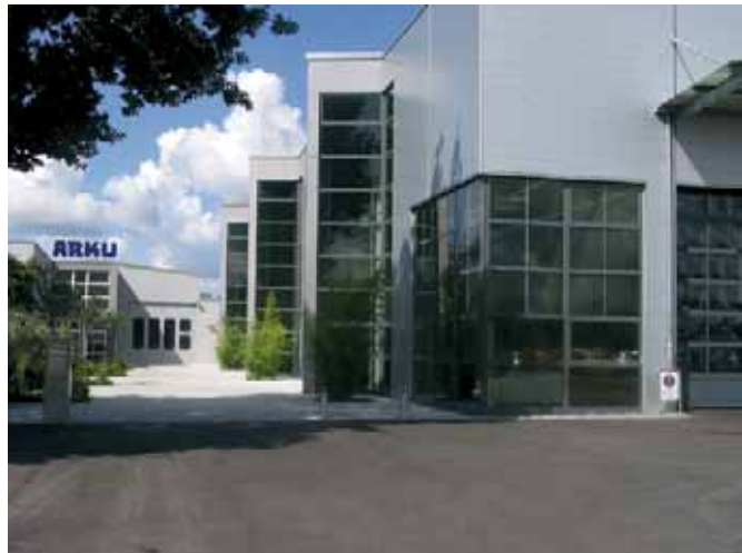
Headquarters and production plant of ARKU GmbH in Baden-Baden/Germany
